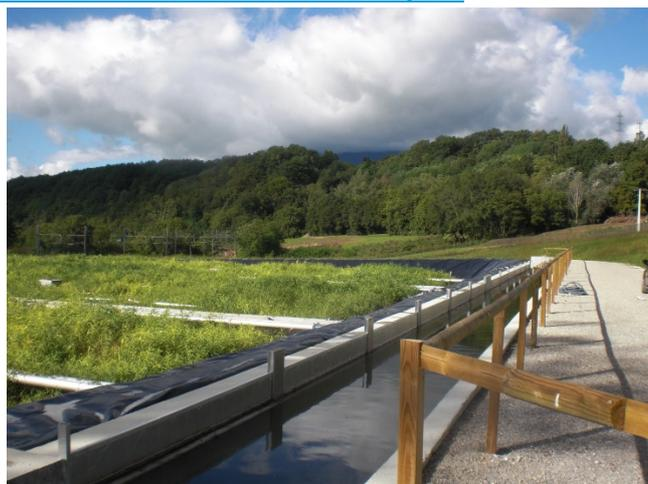
The Challex Vertical flow system (French system) designed for 2,000 PE by SCIRPE is in operation since 2010. It has been designed to treat wastewater from a combined sewer covering a 60-ha domestic catchment area. A specific design has been implemented to treat rain events as well.
