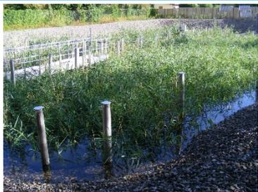
The system is in operation since 2012. It is designed to treat CSO until a hydraulic load of 1,160 m<sup>3</sup>/d while guarantying specific outlet levels for COD, BOD<sub>5</sub>, TSS and TKN. Constructed by Syntea company the system is composed of a vertical flow system (490 m<sup>2</sup>) with a bottom-saturated layer and a controlled outflow structure. The system has been fully monitored during the first four years of operation and used as research site for a PhD.
